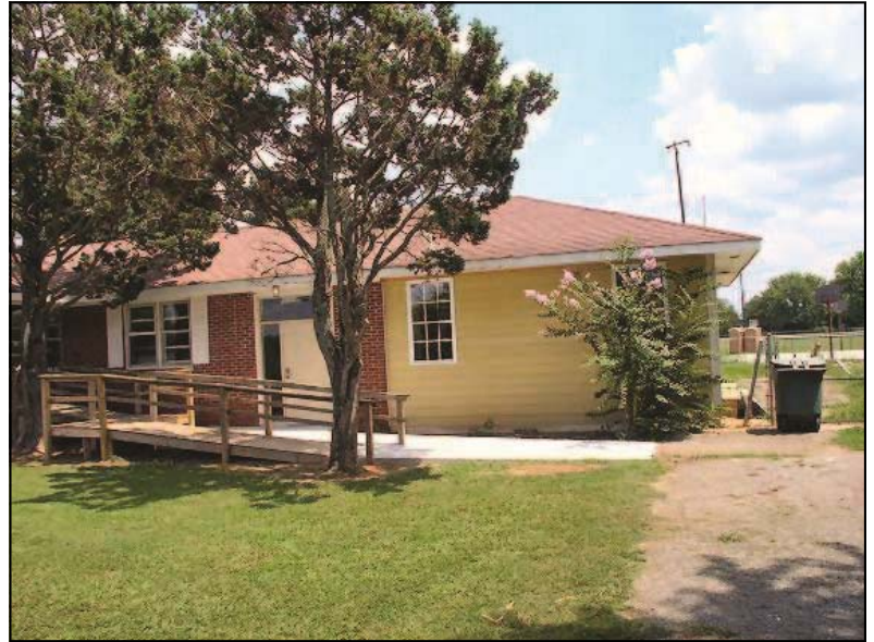
The Madison Crossroads Medical Clinic extends from the doorway between the two brick sections to the end of the house. This was once the carport of the residence. The Huntsville Assistance Program (HAP) occupies the other part of the building.
